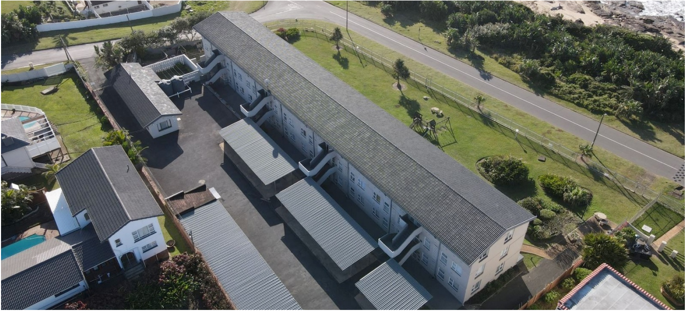
Jacaranda Holiday Flats in Uvongo, KZN. The entire roof was re-roofed with Harvey EcoTile® for a lightweight, corrosion resistant and low maintenance solution.
